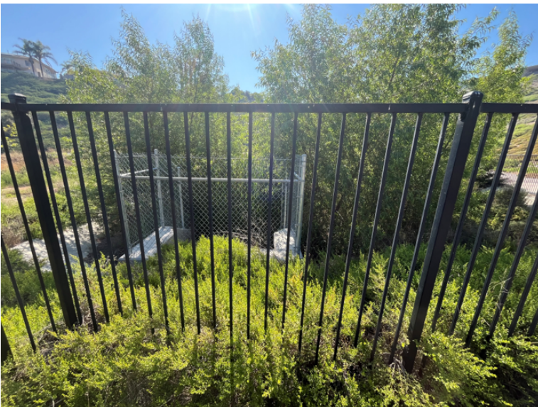
Before & After Drainage Channel Clean-Out.
